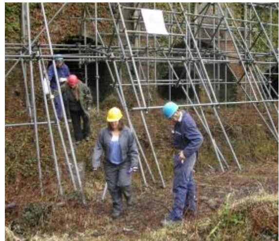
Brockham Lime Kilns. Photos, Derek Smith.
